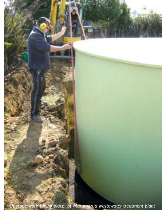
Upgrade work taking place at Maramarua wastewater treatment plant
